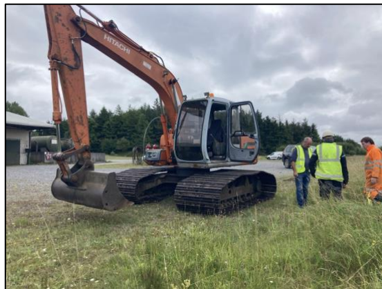
View of location of Infiltration Pit 5a
