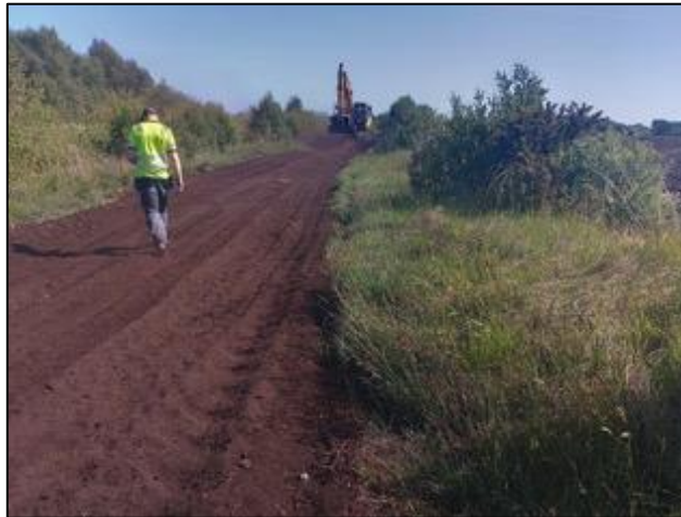
Plate 8: View of location of TPC05 prior to excavation.
