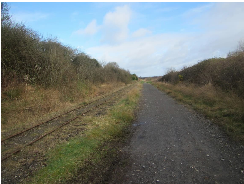
Plate 8.14 Route of the 220kv buried cable following track and railway line.
