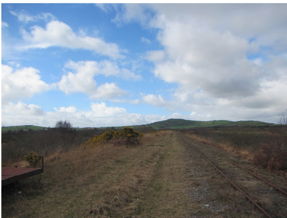
Plate 8.12 Route of the 220kv buried cable with Croghan Hill in the background.
