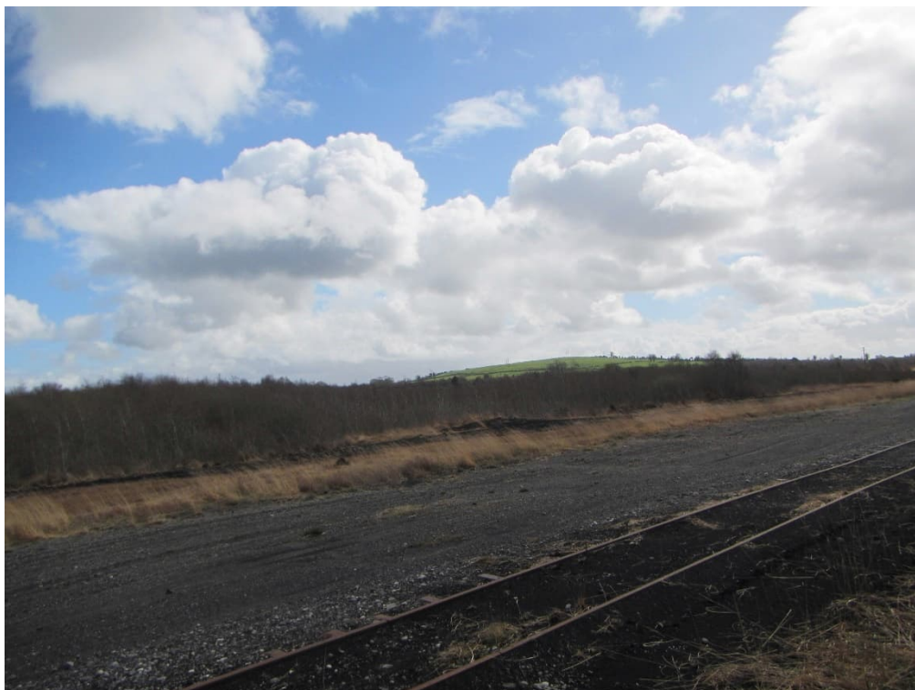
Plate 8.11 Overhead Connection Route – Looking towards Clonin Hill.
